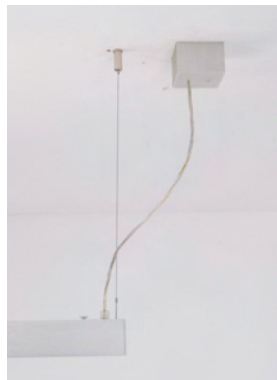
Cubicolo / ceiling box
